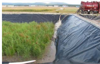
Application of sludge to sludge cell
